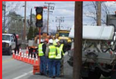
Roadside Utility Repair
